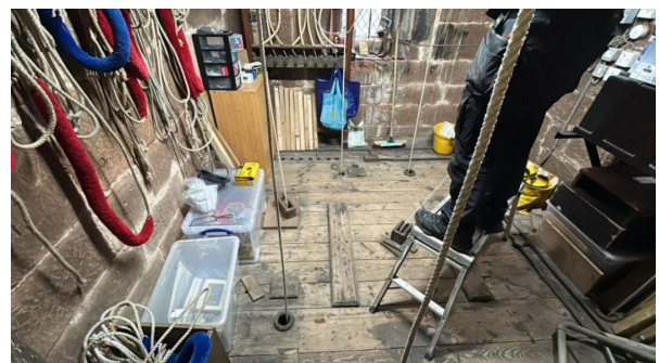
View from middle room with new LED batten:
